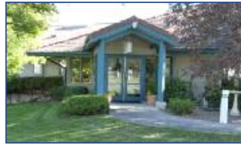
Current North Building Entrance.
