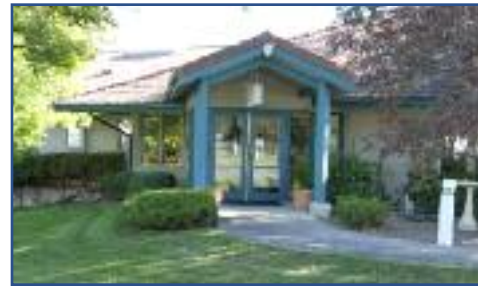
Current North Building Entrance.
